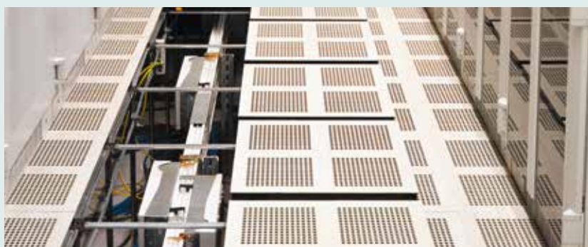
The construction of the individual server rooms (cages) represents a major technical challenge. Here, fire protection must be integrated into elevated (so-called raised) floors in conjunction with lightweight stud wall constructions. Photos: © www.lindner-group.com
