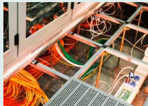
The construction of the individual server rooms (cages) represents a major technical challenge. Here, fire protection must be integrated into elevated (so-called raised) floors in conjunction with lightweight stud wall constructions. Photos: © www.lindner-group.com
